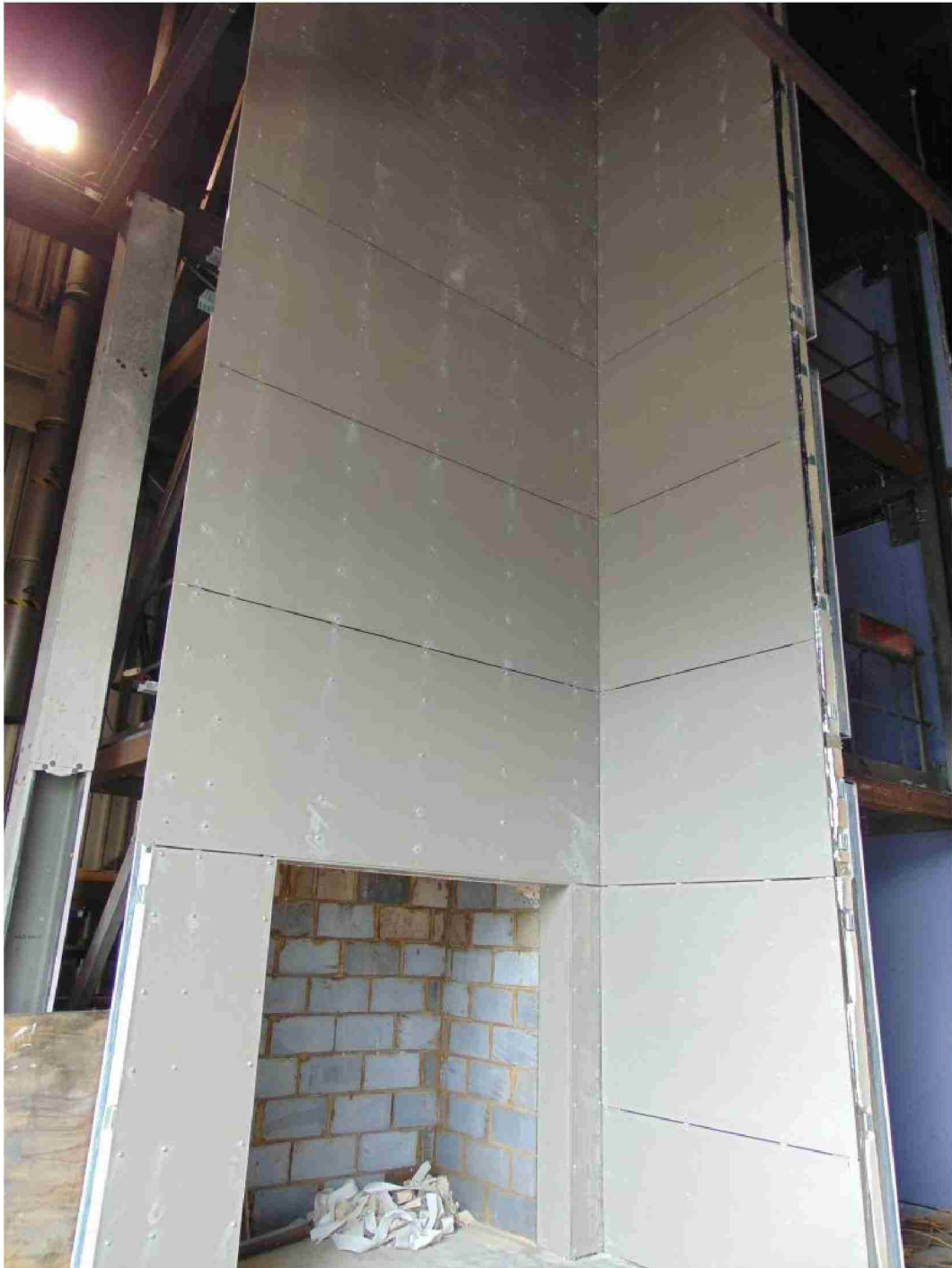
Figure 1. Full-height view of complete system prior to test.
