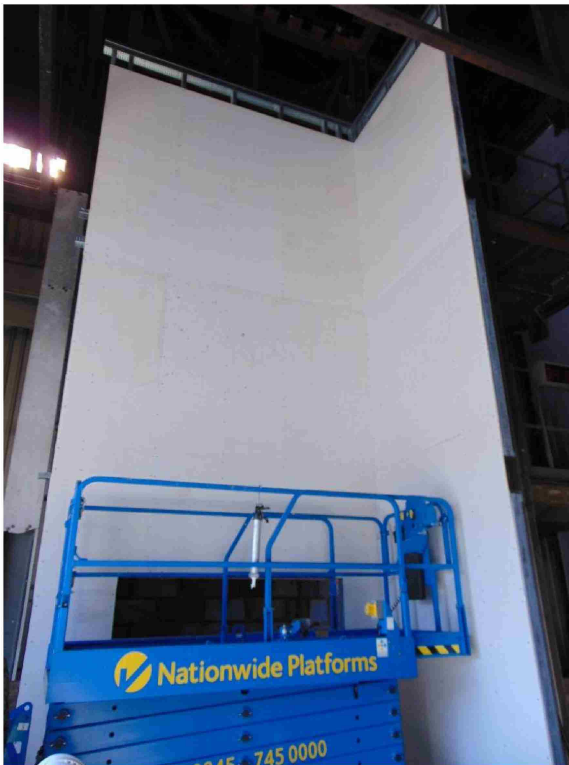
Figure 5. Full-height view of sheathing board layer.
