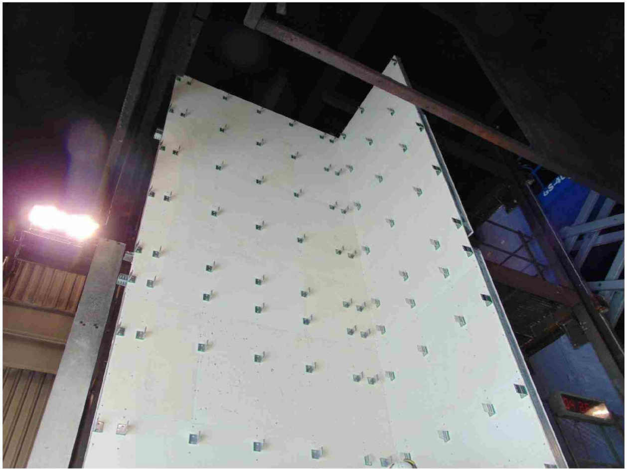
Figure 8. 'L'-shaped helping hand brackets fitted to the sheathing board.
