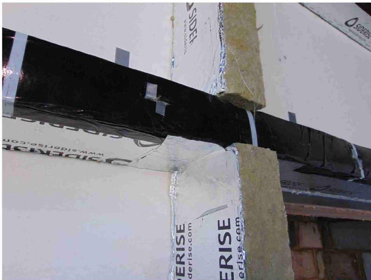
Figure 7. Junction between horizontal and vertical cavity barriers.
