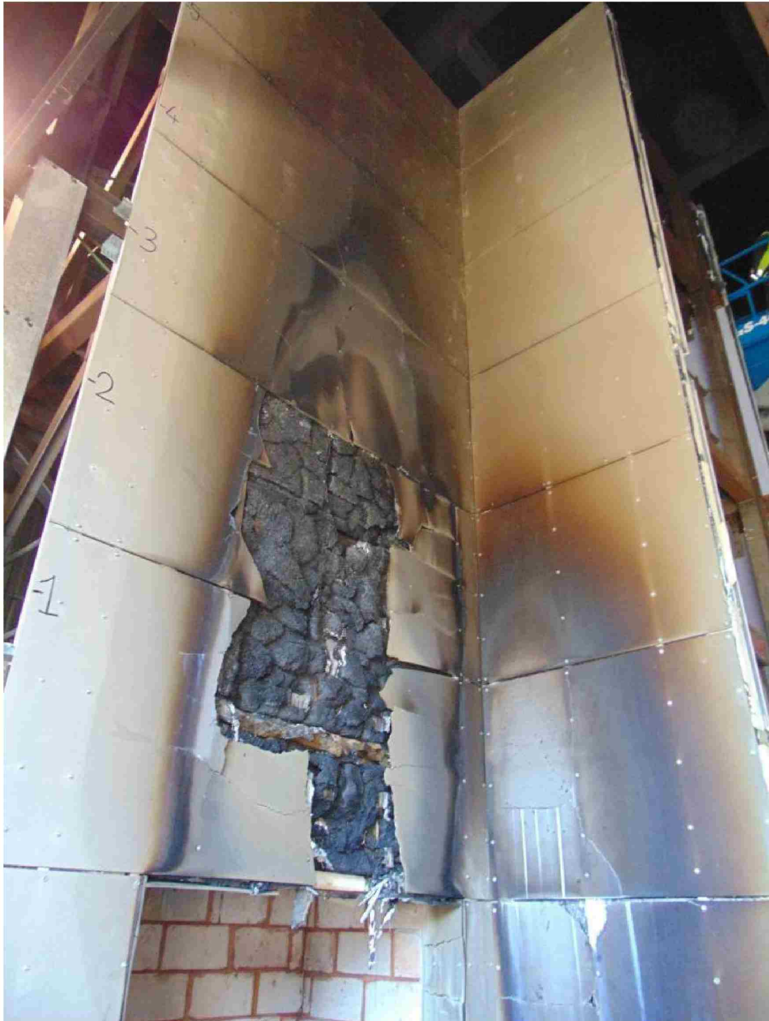
Figure 25. Post-test view of tested system from the top of the combustion chamber to the top of the cladding system.
