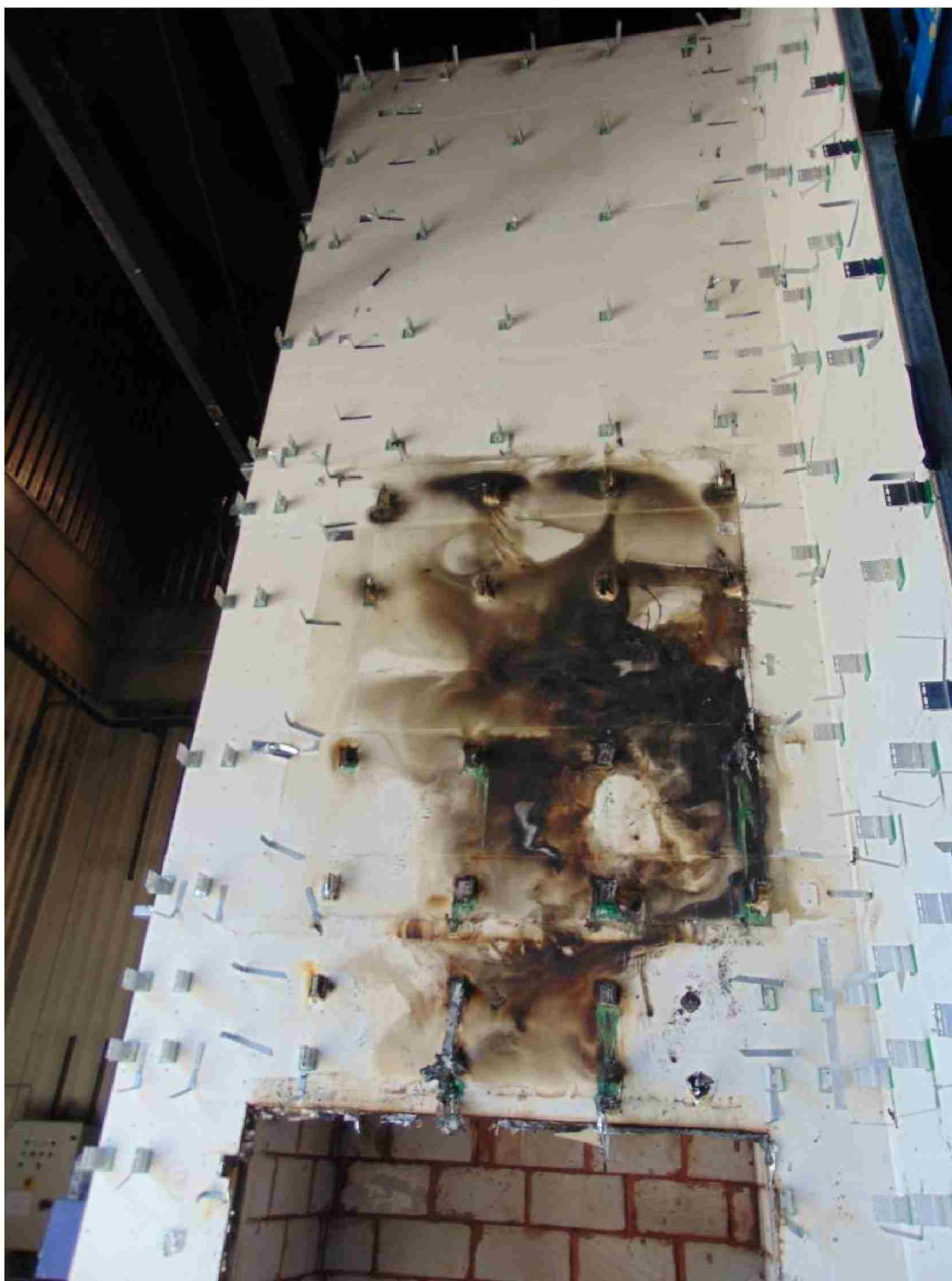
Figure 30. Post-test main wall view of sheathing board and brackets from the top of the combustion chamber to the top of the cladding system.
