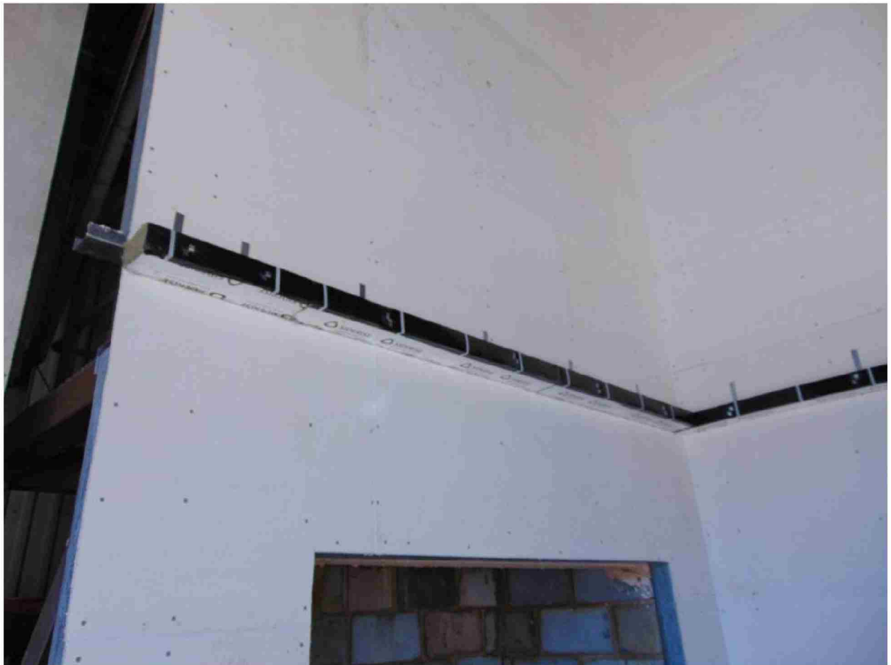
Figure 6. Second row of horizontal cavity barriers installed.
