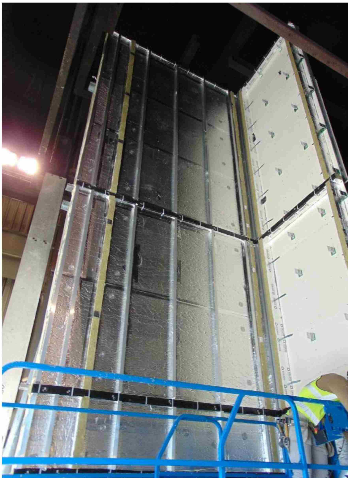
Figure 9. Insulation, cavity barriers and rail substructure fitted to the main wall.
